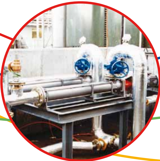
Pumping of slurry mix
